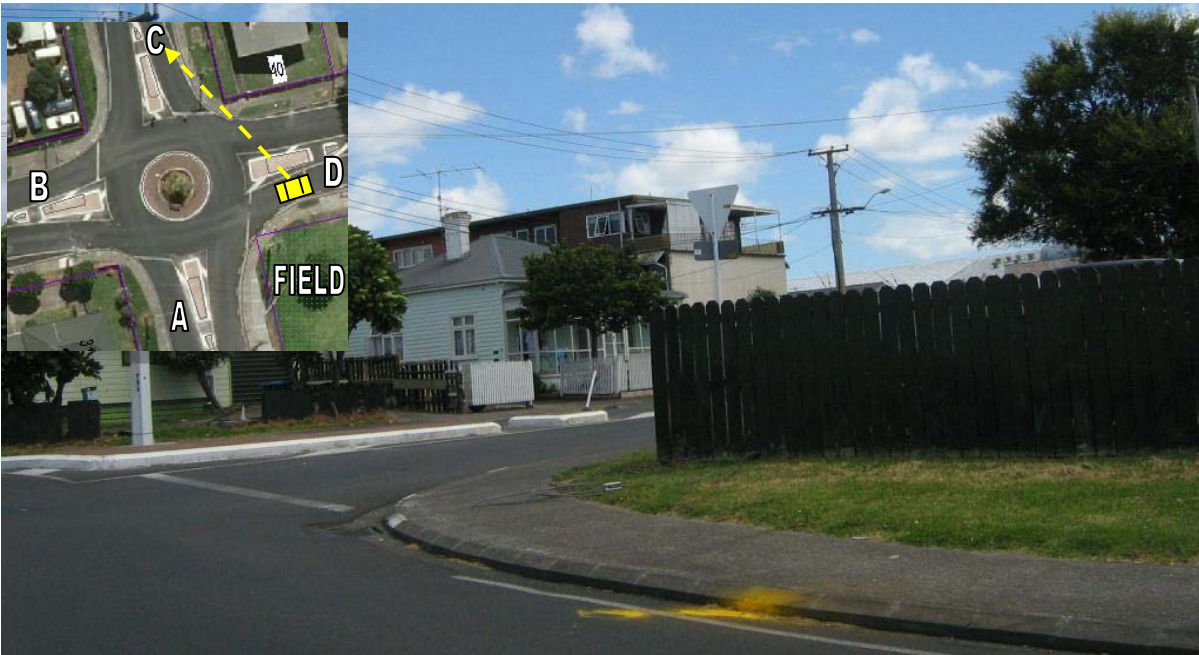
FIGURE 5: Example photo taken 10 m (33 ft) back from the limit line on approach D to the small Church Street / Avenue Road roundabout in Otahuhu, Auckland. Sightline restrictions are almost identical for approaches B-D, whilst approach A has virtually unimpeded visibility due to the presence of a field on the right.
