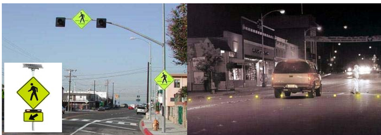
FIGURE 1: Flashing road sign (left) and road stud (right) installations in the US, with the more recently developed RRFB shown inset left.
