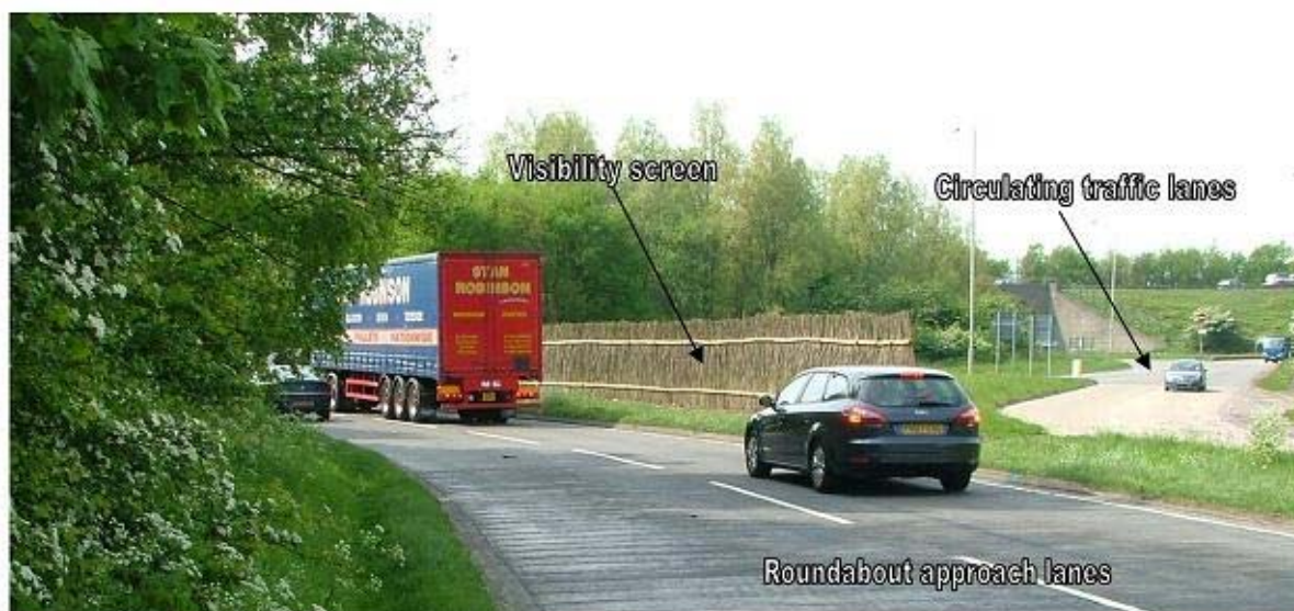
FIGURE 4: Photo taken in 2008 of a 2.5m (8 ft) high visibility screen installed on the approach to a roundabout at the intersection of the A50/A511 and Junction 22 of the M1 motorway in Markfield, Leicestershire County Council, UK.
