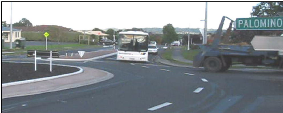
Figure 7: Photo showing a bus straddling both lanes whilst waiting at the roundabout limit line to turn right.
