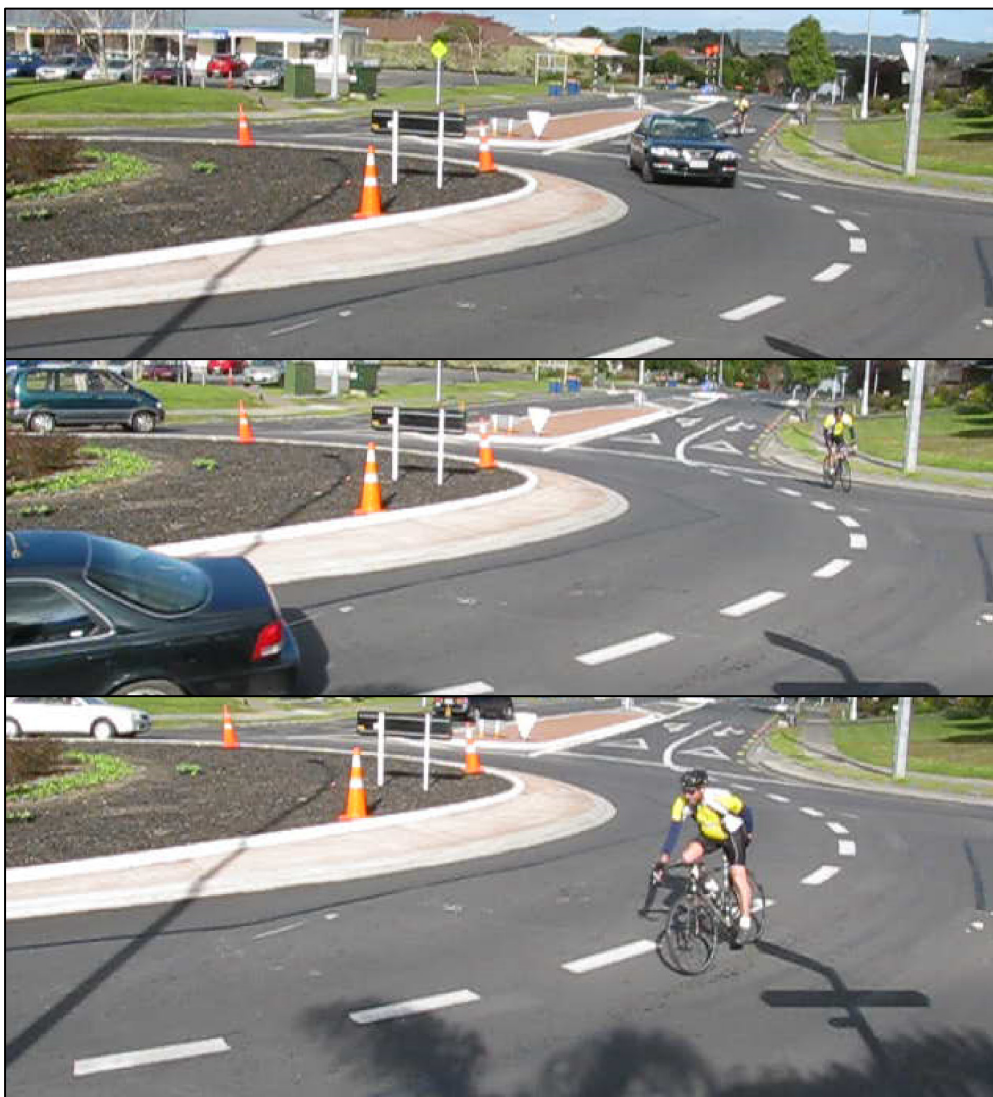
Figure 8: Photos showing a cyclist travelling through the C-Roundabout using the middle of the traffic lane as desired.
