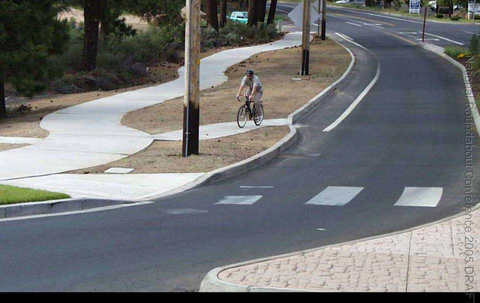
What if a cyclist doesn't want to enter the roundabout? Provide a ramp at busy roundabouts
