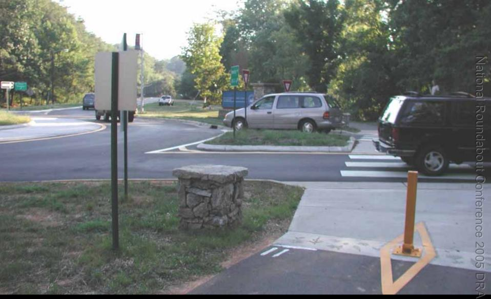
Crosswalk Placement – 20' back from edge line – provides gap between queued vehicles
