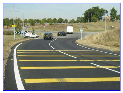
Figure 46: Transverse Yellow Bar Markings at Roundabout Approach
