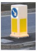
Figure 45: U.K. Style Internally Illuminated Bollard
