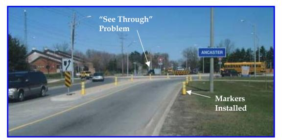
**Figure 8**: Ancaster Roundabout with Candlestick Bollards on EB Approach (Note "see through" problem of central island)
