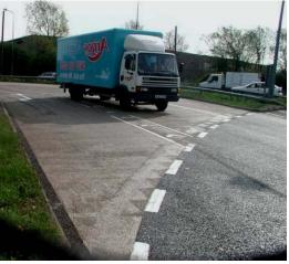
Figure 16 - Shell-coat Skid Treatment
