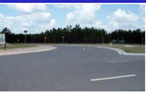
Two Lanes Merge into one within a roundabout from both left and right create a free-for-all that forces drivers to merge while traveling a double reverse curve
