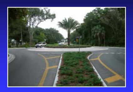
Good drivers can pass through a 23 mph designed roundabout at 27 mph and more than 30 mph through a roundabout with 25 mph design speed. I prefer to limit all of my roundabouts to 23 mph or less to truly limit vehicle speeds and reduce the lowest crash rates
