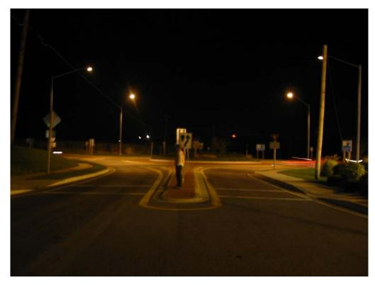
symmetrically around the roundabout as shown in Figure 2. It provides a good illustration of uniform lighting of the circulatory roadway.
