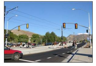
The author was involved in the analysis and design of a roundabout at the University of Utah that included light-rail crossing through the center and a pedestrian crosswalk signal on one of the three legs. See photos below. The crosswalk signal creates serious backups into the roundabout during peak traffic flows that impact one exit of the roundabout. The crosswalk is a mid-block location approximately 150 ft. from the exit of the roundabout.
