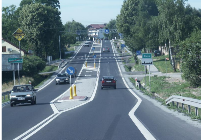
FIGURE 1 View of the beginning of the model road section. Cross-section with additional multifunctional median lane
