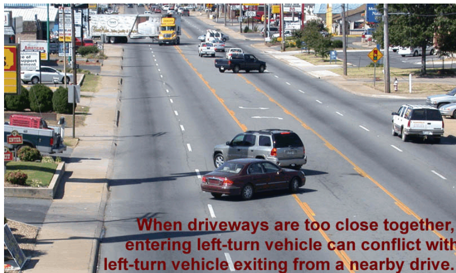
EXHIBIT 3-10 One of the many problems that results from driveways too close together
