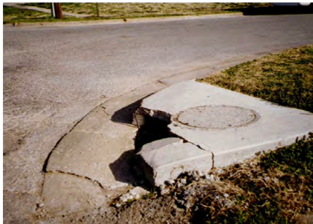
EXHIBIT 3-38 Inadequate radius
