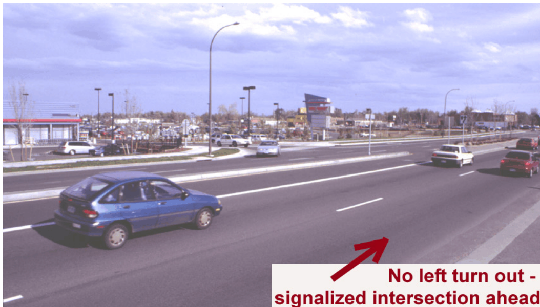
EXHIBIT 3-23 Partial median opening allows only left turn into the site
