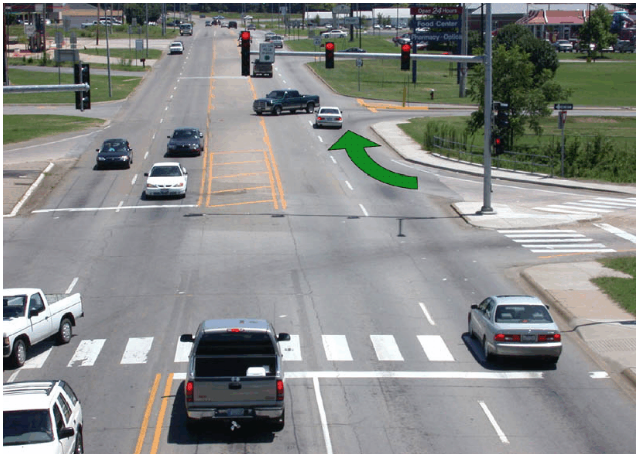
EXHIBIT 3-18 Traffic conflict with close spacing at ramp-crossroad junctions
