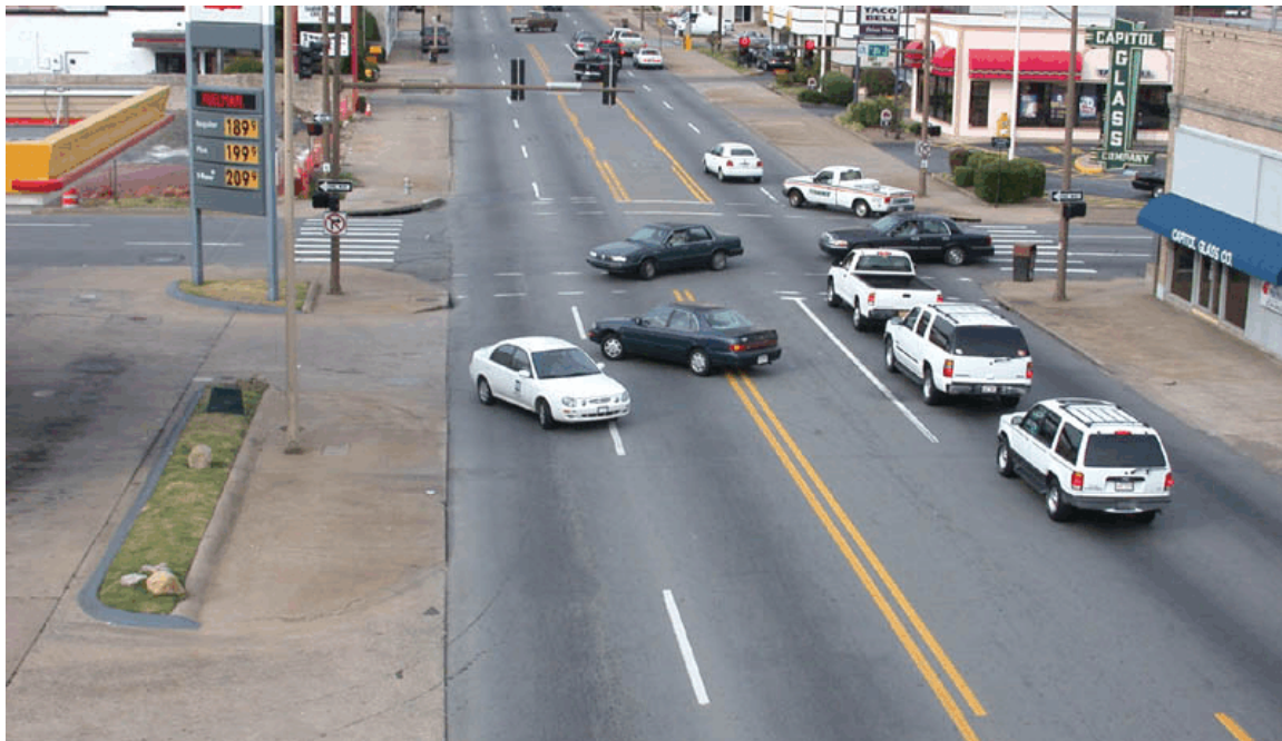
EXHIBIT 3-14 Conflicts arise from inadequate corner clearance
