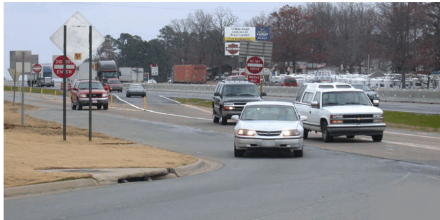
EXHIBIT 3- 8 Frontage road-street intersection too close to upstream exit ramp
