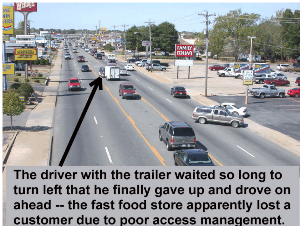
EXHIBIT 2-40 A TWLTL does not always guarantee quick access
