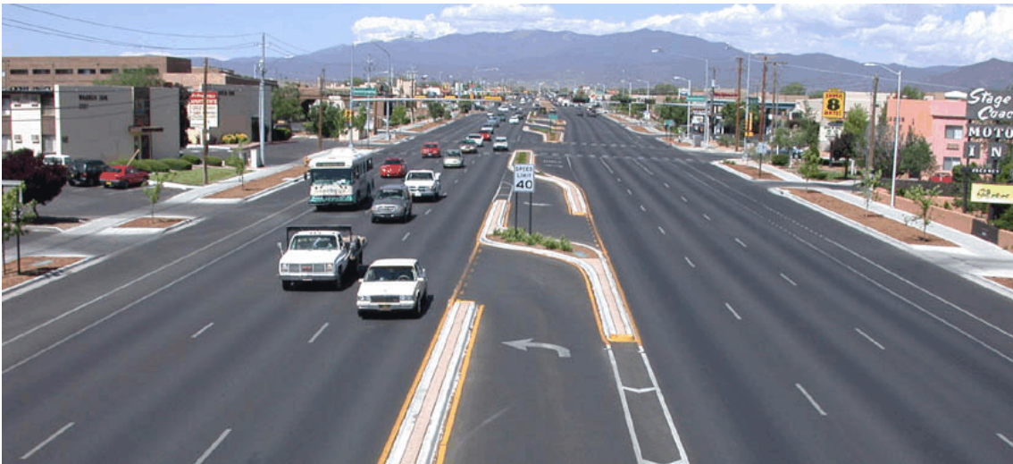
EXHIBIT 3-47 Example corridor retrofit
