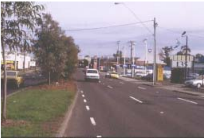
Direct commercial frontages can reduce arterial road efficiency and safety.
