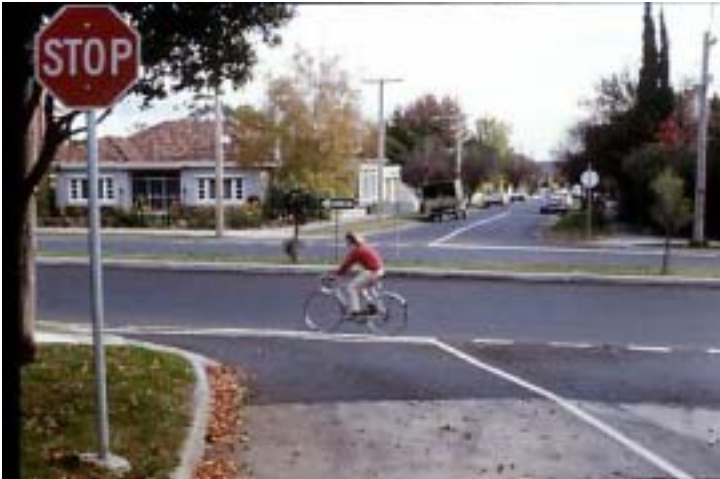
Medians across minor junctions can control right turns into and out of local streets.
