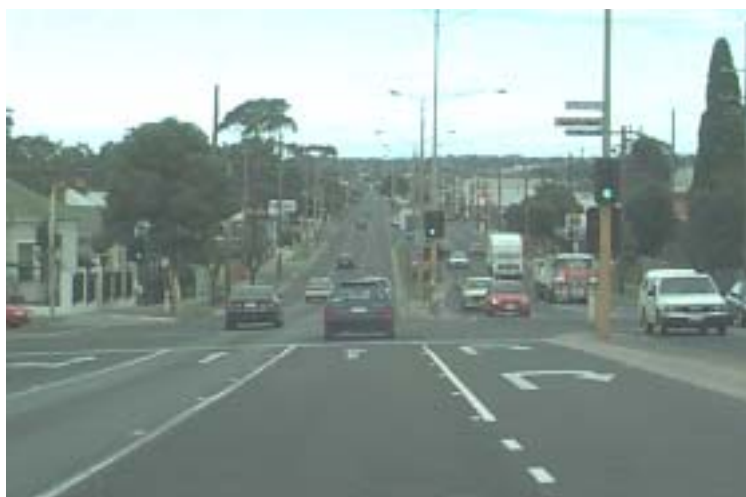
Medians control where right turns and U-turns can occur.
