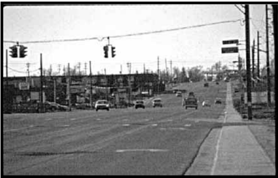
Figure 4: South Golden Road prior to reconstruction (5).
