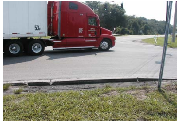
Truck makes wide swing into on-coming traffic lane. Note shoulder rutting from tracking of rear wheels of trailers.
