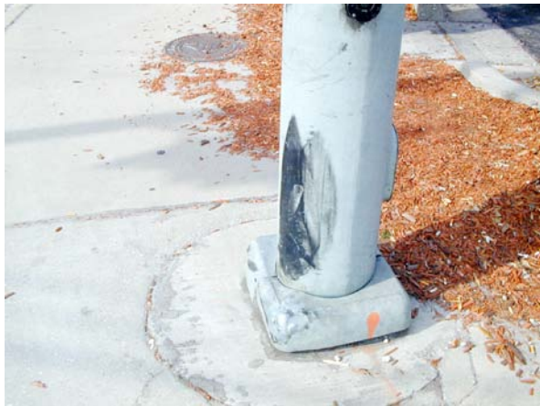
Sidewalk and infrastructure damage resulting from insufficient turning radii and the location of utilities infrastructure.
