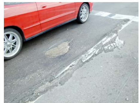
Rutting and heaving deterioration caused by heavy trucks.
