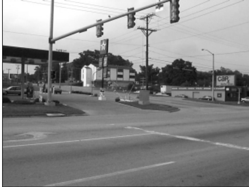
Figure 24—Inadequate corner clearance: safety and operational concern
