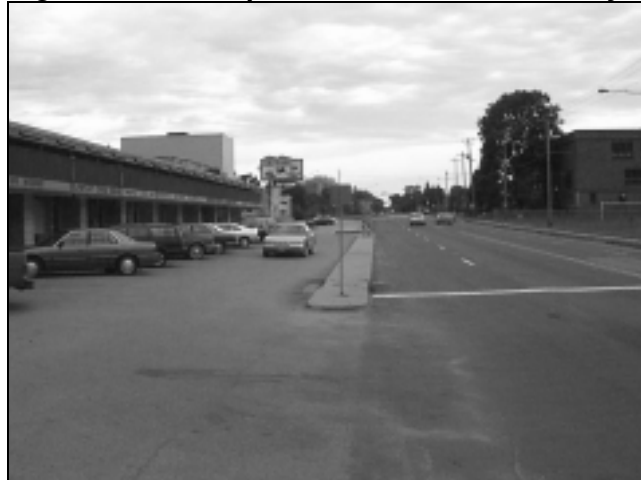
Figure 41—Example of insufficient driveway throat length
