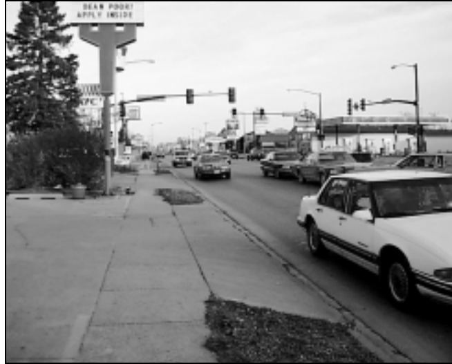
Figure 22—Inadequate driveway spacing
