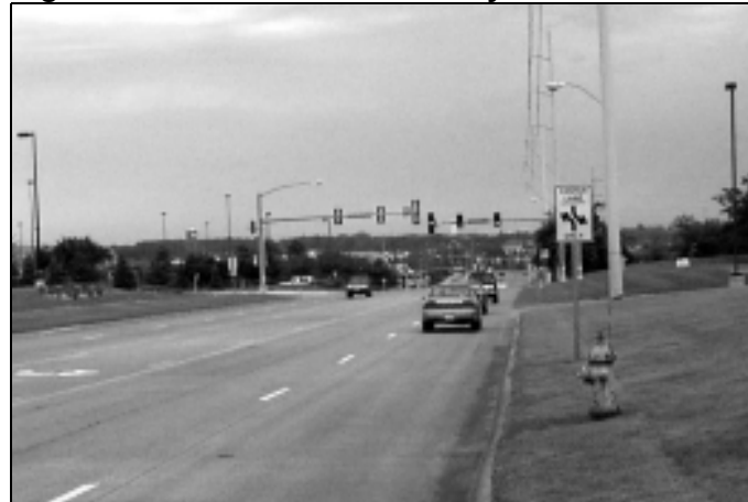
Figure 50—Continuous two-way left turn lane
