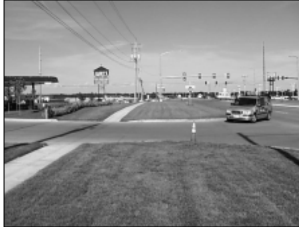
Figure 25—Good corner clearance and large lot to accommodate high volume use (traffic signal indicates location of intersection)
