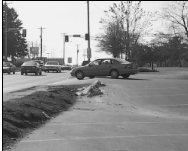
Figure 37—Driveway slope: Steep slope forces motorists to unduly reduce speed to negotiate driveway. This vehicle is almost “bottoming out.”
