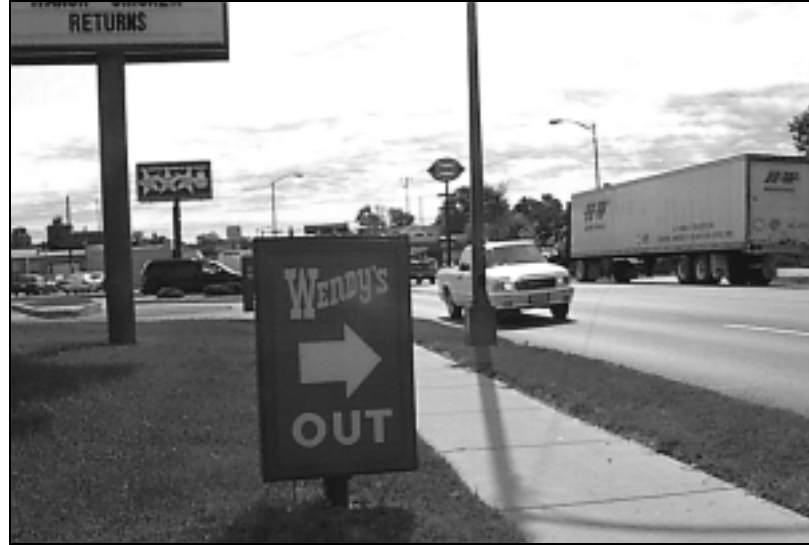
Figure 19—Inadequate sight distance (viewed from a driveway)
