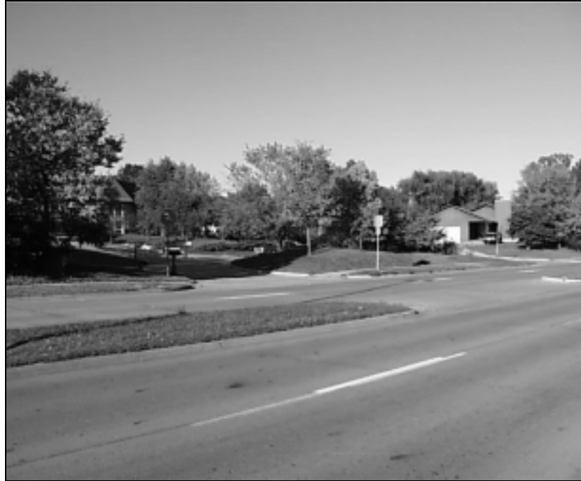
Figure 28—Internal access roads
