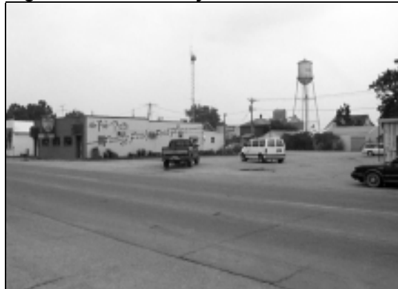
Figure 36—Driveway width: unrestricted access creates potential safety concern
