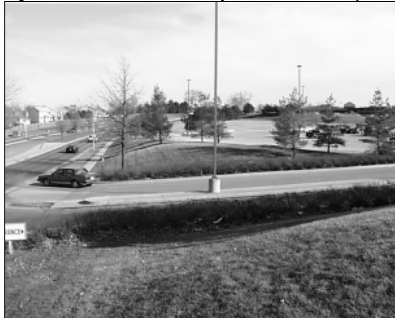
Figure 42—Commercial driveway with wide landscaped buffer
