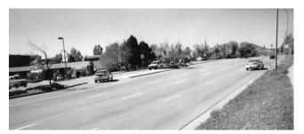
*Figure 16. Directional median opening at three-leg intersection.*
