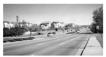
*Figure 17. Conventional median opening at four-leg intersection.*
