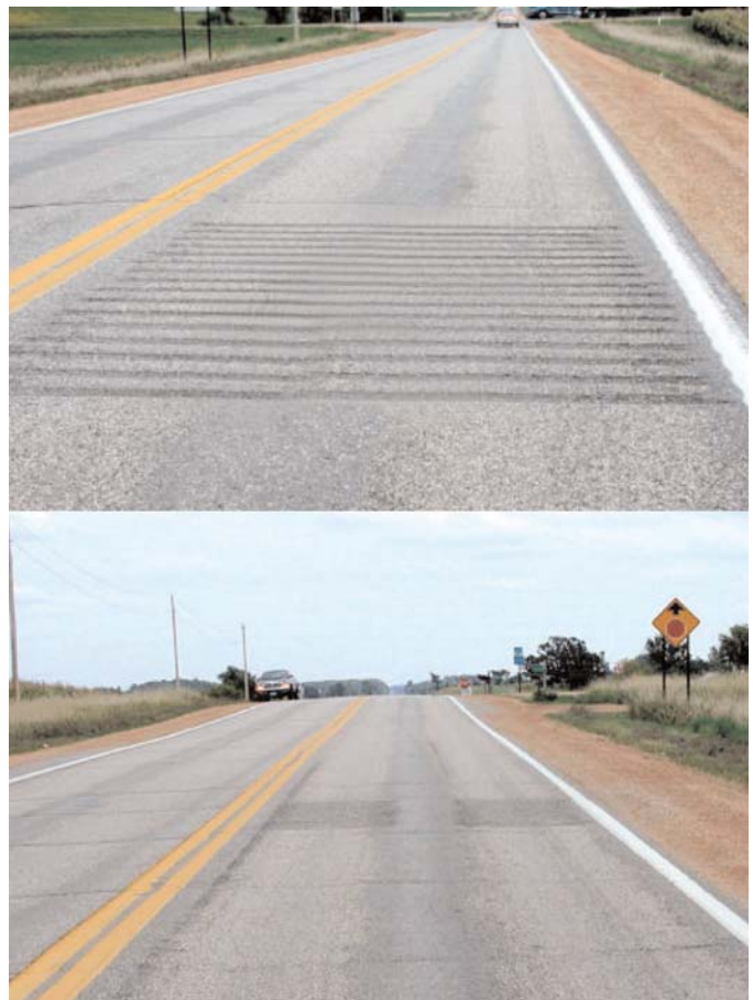
Figure 45. In-lane intersection approach rumble strips (59).
