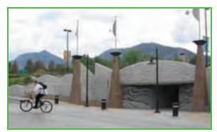
Boulder reconstructed the approach and facade of this underpass connecting off-campus student housing to the main CU campus. The project set back the opening to improve site distance and installed a raised intersection crossing of the road. New artwork celebrates this gateway to the campus and makes the underpass inviting to users.
