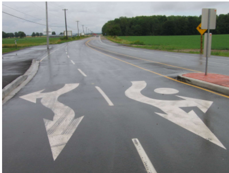
Photo: Ourston Roundabouts Canada
