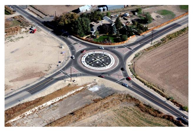
FIGURE 5 Happy Valley and Amity - constructed initial-build single-lane roundabout (looking northeast).
