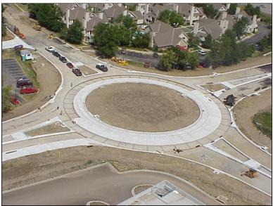
Figure 5: Construction sequence consisted of placing the concrete for the inner ring of the circulating lane first followed with half of the middle ring. The remaining half of the middle ring and half of the outer ring is being formed. Note the monolithic curb and pavement sections on the splitter islands and outer curb line.
