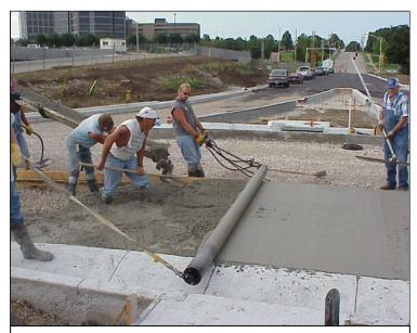
Figure 2: The concrete was placed between the concrete curb of the internal island and wooden forms and a roller screed was used to provide the initial finish of the circulating lanes. Both of the edges the roller screed rested on had to be kept clean to ensure a smooth finish.
