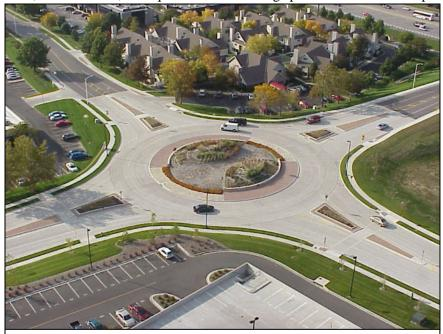
Figure 1: Photograph of the completed concrete roundabout, looking northnorthwest. The conference center is in the foreground. Note the two vegetated berms in the central island, behind the retaining walls.
