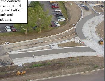
Figure 6: Placement of the concrete in the remaining half of the outside ring of the circulating lanes occurred simultaneously with some of the approach and departure lanes. The concrete pavement ended at the end of the splitter island. The pavement approaching the roundabout was asphalt, except on the east leg which was totally concrete.
