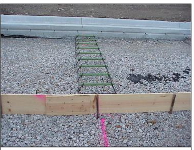
Figure 3: The joint pattern was spray painted on the aggregate base and projected from inside to outside curb to ensure the joints lined up across the circulating lanes. This also provided a guide for placement of the dowel bar baskets.
