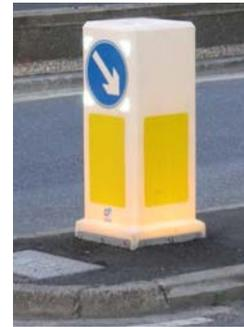
**Figure 45:** U.K. Style Internally Illuminated Bollard
