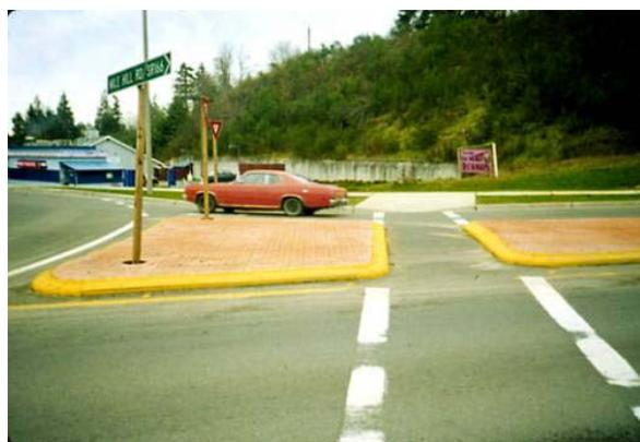
Figure 11 - Cross Walk Alignment That Is Too Enticing
