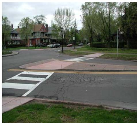
Figure 9 - Poorly Located Cross Walk
