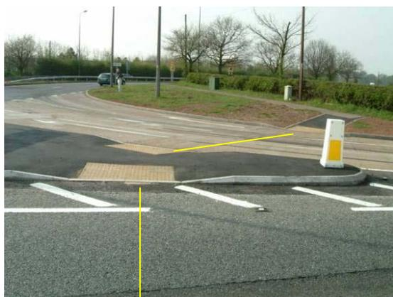
Figure 10 - Angled Cross Walk with Detectable Treatments
