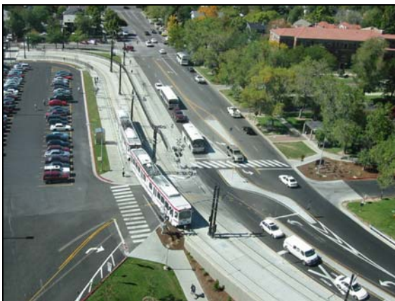
Side-running to Center-running Transition Point
