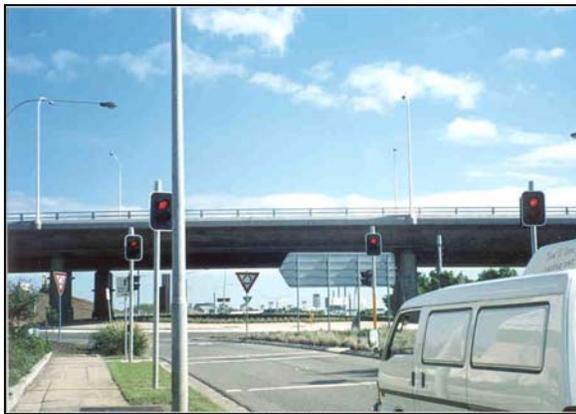
The roundabout interchange with flyover at Homebush Bay replaced an at-grade roundabout at the same location before the M5 Motorway and Flyover were constructed. Because of several hundred pedestrians crossing this location during the 2000 Summer Olympics from a nearby train station the pedestrian crosswalk signal was clearly warranted.
