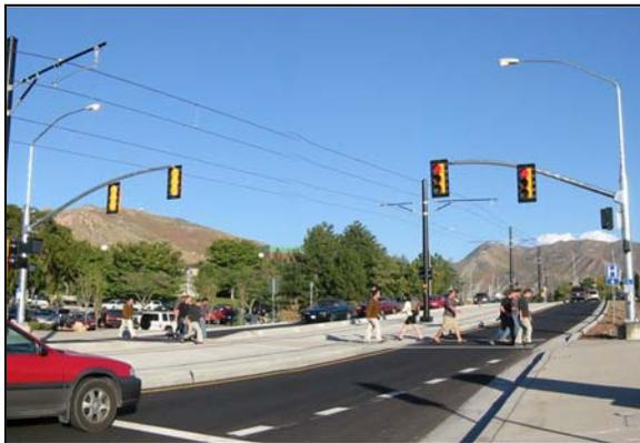
The author was involved in the analysis and design of a roundabout at the University of Utah that included light-rail crossing through the center and a pedestrian crosswalk signal on one of the three legs. See photos below. The crosswalk signal creates serious backups into the roundabout during peak traffic flows that impact one exit of the roundabout. The crosswalk is a mid-block location approximately 150 ft. from the exit of the roundabout.
